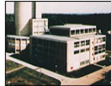
AVR, Germany 15 MWe, 1967-88
