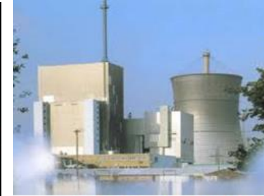
THTR, Germany 300 MWe, 1986-89
